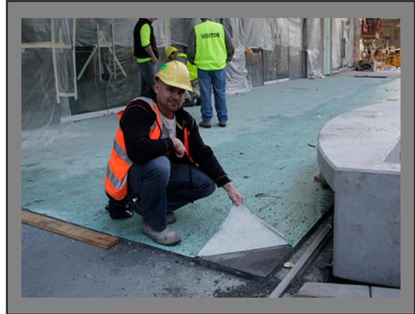
**External Weather Resistance** - The Floordefend system offers protection for up to 9 months externally.
