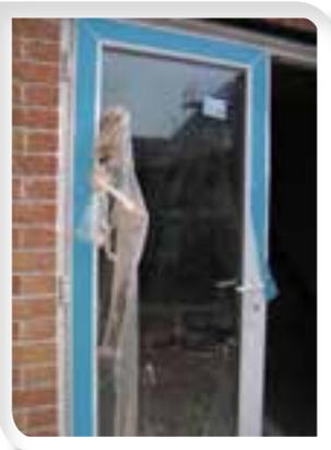
Spraylat do have many construction companies enquiring about Protectapeel after using traditional protective film on rolls. The general consensus is that the traditional films just peel away from the surface during the construction project - as you can see in this image the film has parted from the surface, damaging it causing additional cleaning costs or even worse replacement costs.
