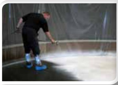
Protectapeel is applied directly to the floor to temporarily protect it from construction site damage. Available in grey as standard or clear or pigmented with a colour upon request.
