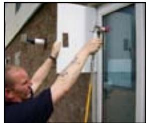
**2.** Point the nozzle at the area you wish to protect and hold the spray gun 300- 400 mm from the substrate. Use the Protectapeel shield to prevent overspray.
