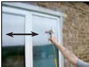
**3.** Release the safety catch and start spraying in a horizontal direction. Keep the gun at right angles to the surface. This means moving your entire arm back and forth rather than flexing the wrist.
