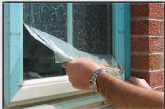
*Simply hand peel Protectapeel away - taking all the site dust with it, leaving you with clean and undamaged surfaces.*
